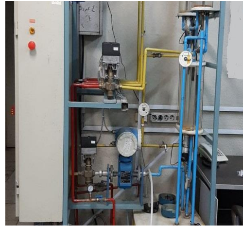
Fig. 1. A schematic of quadruple tank located in Faculty of Electrical Engineering at K.N.Toosi University
